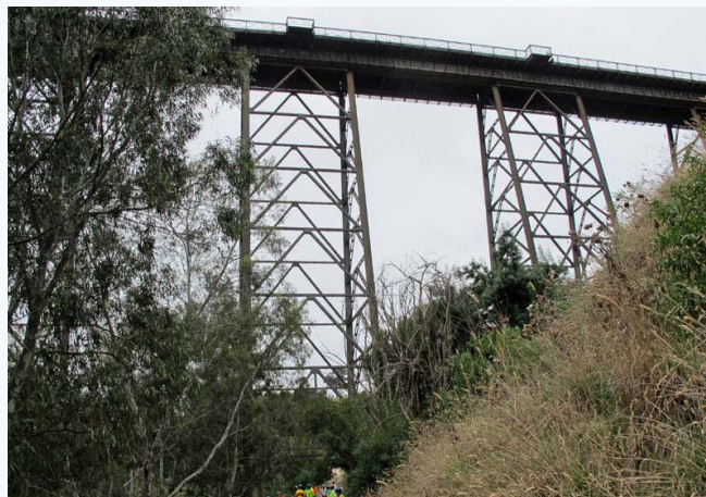
The railway trestle bridge across the Maribyrnong.
