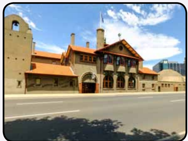
View towards Mission to Seafarers Victoria from Seafarers Bridge, with redevelopment work underway.
