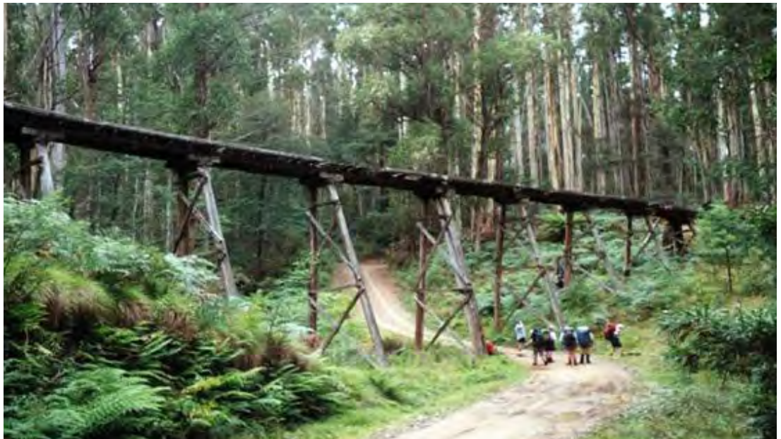
Old trestle bridge, Upper Rubicon
