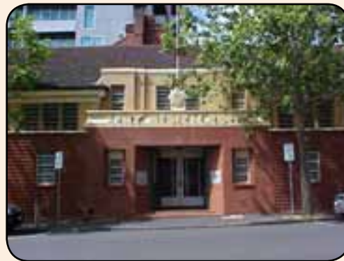
RHSV entrance on A'Beckett Street
