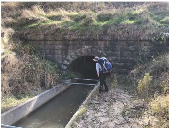
Fine stonework on the old tunnel entrance
