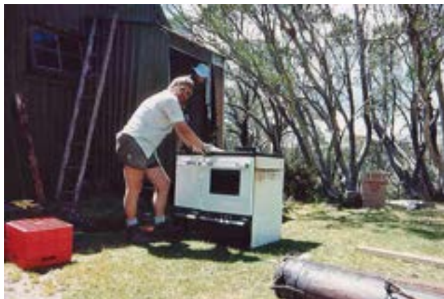
Helping to install a new stove at Wilky
